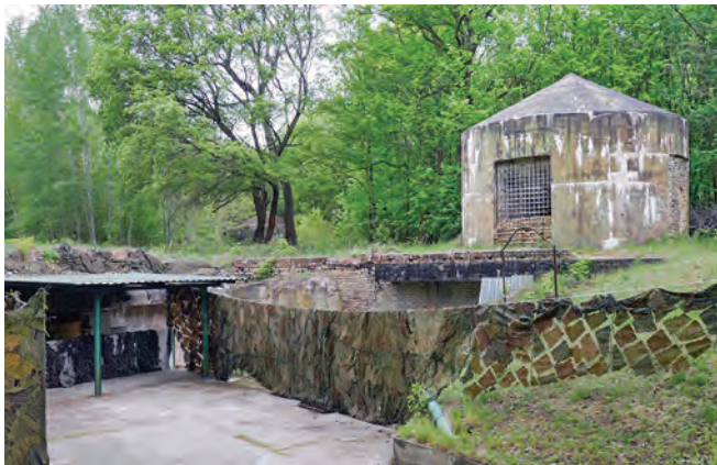
Hardened airshaft and emergency exit of Zeppelin/Ranet. Photo Vin Stenhouse
